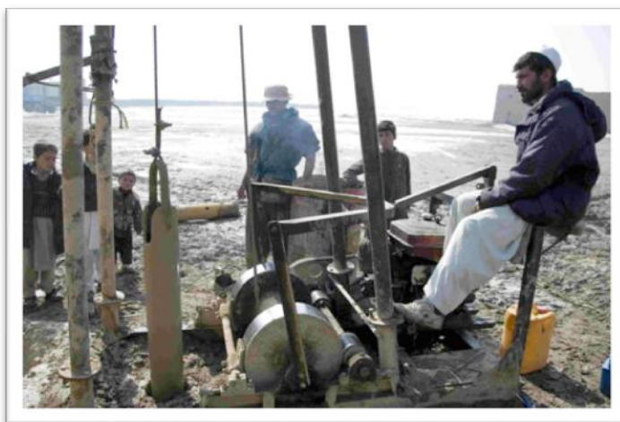
Construction of a water point in Shakadara, February 2007.
